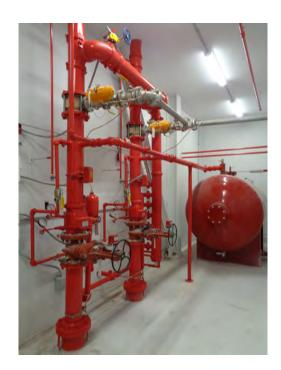
It is most important that the foam concentrate is fed into the ratio controller at a pressure which is similar to the water pressure as it enters into the same ratio controller. This is accomplished by using either a Bladder Tank or a positive displacement foam pump with any In-line Balanced Pressure Proportioner (ILBP.)
